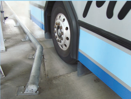
Galvanized guide rails use a 'rolling' design, preventing buses from climbing out, to keep the wash running smoothly
